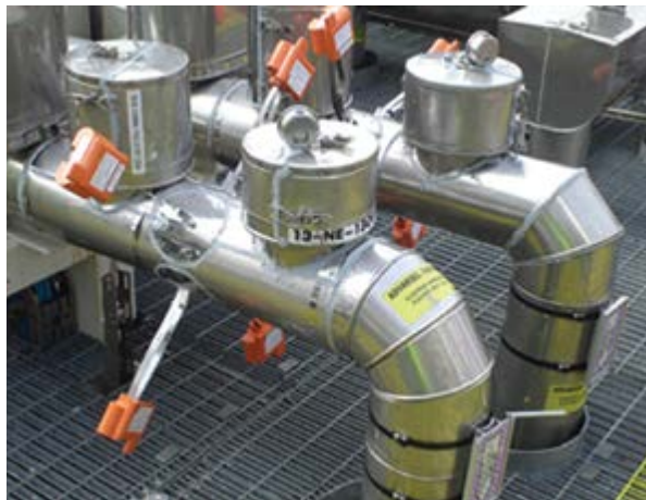
Figure 2. Installing multiple ultrasonic units (orange) in areas at elevated risk of internal corrosion can help spot localized attack.
