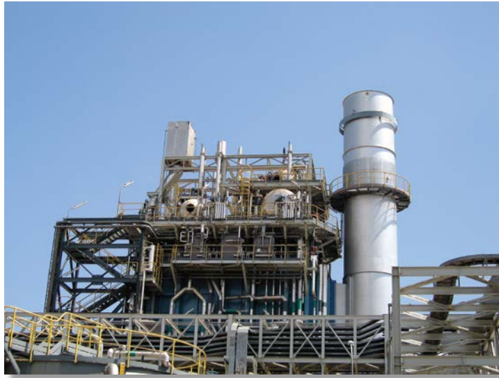
Fig. 1. Pressure safety systems are essential for safely operating processing plants.
