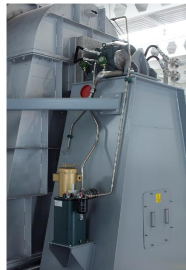
Figure 7. Hydrodynamic fan bearing configured for circulating oil.
